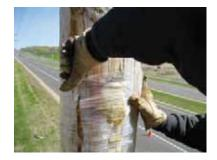
Remove all debris and water from the hole. Duct putty may be used to fill any cracks at bottom of the hole to prevent UPR Pole Repair<sup>™</sup> from leaking out.
