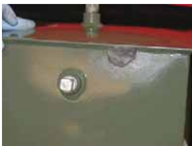
Apply putty ½ inch beyond leak; ⅛ to ¼ inch thick
