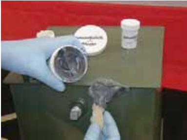
Apply PowerPatch® Sealant over putty patch or leak area
