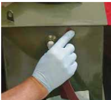
Sand or brush repair area
