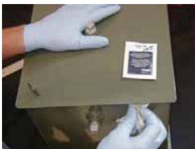
Clean area with Type TR™ before applying PowerPatch® Putty
